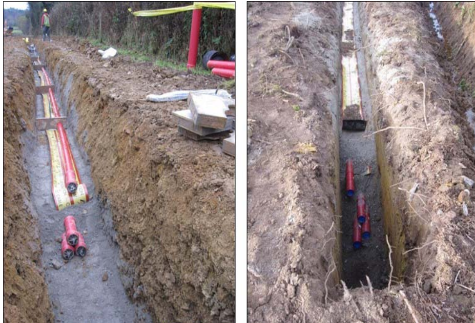
Plate 2.1 Cable Trench View
