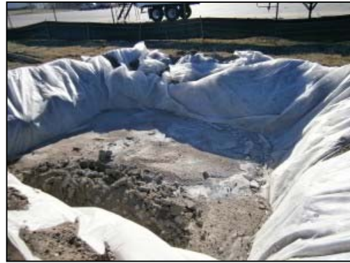
Plate 3.2 Concrete washout area
