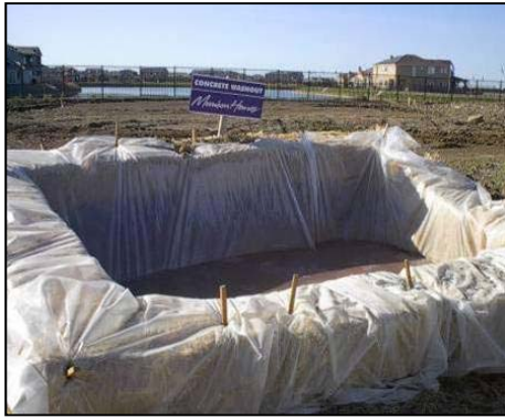
Plate 3.1 Concrete washout area
